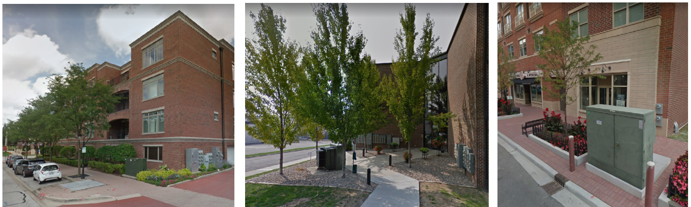
Figure 7-T. Examples of Poorly Located Utility Appurtenances on Primary Streets: NOT PERMITTED
