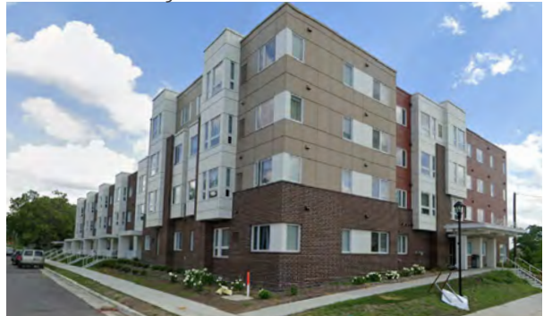
General Building on Blake Road
