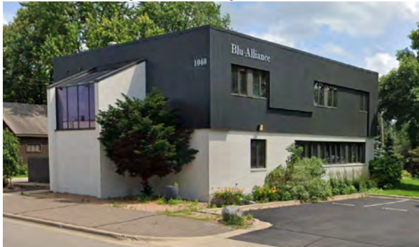
General Buildings in the Neighborhood Centers
