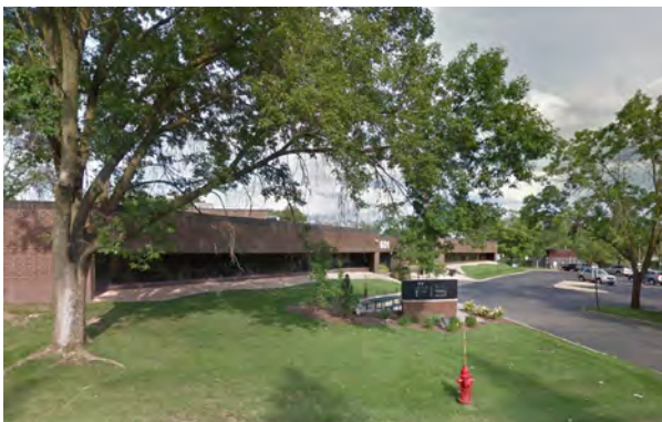
Suburban General Buildings in Hopkins
