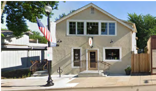
Commercial Cottages and a Storefront Building on West Mainstreet
